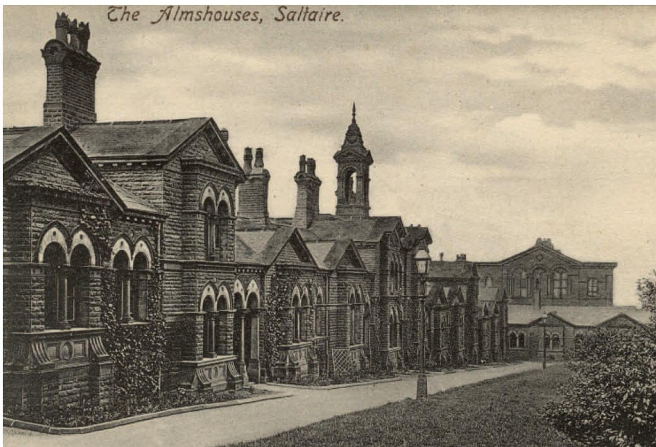
Illustration 4: Early postcard image of Saltire Almshouses on west side of Victoria Rd (showing now demolished Saltire Methodist Chapel in background)
