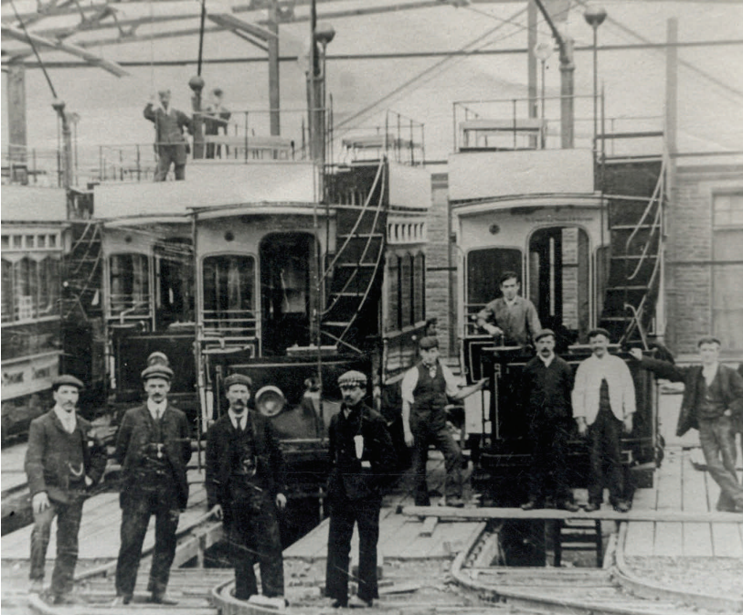
Saltaire Road tramsheds in operation
