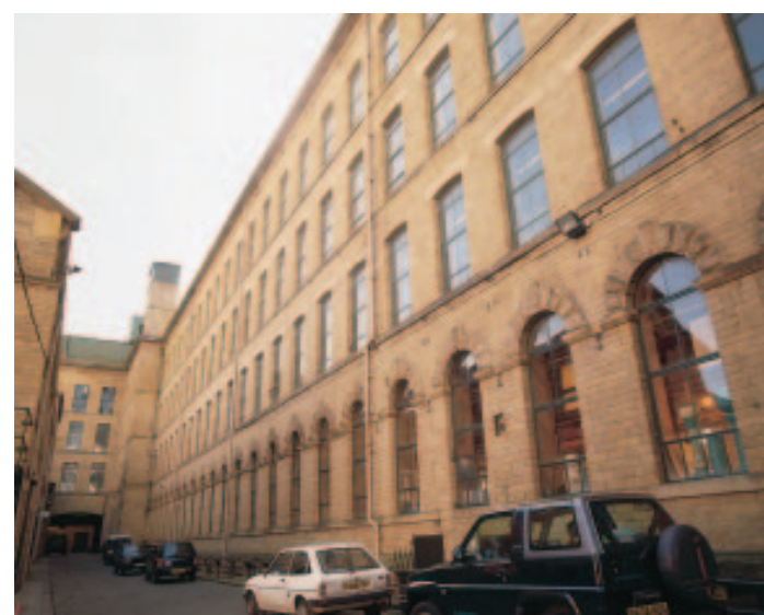
The elevation shows the north face of the main spinning mill from the inner mill yard which retains its stone setted carriageway. Original cast iron window details survive on the mill.
